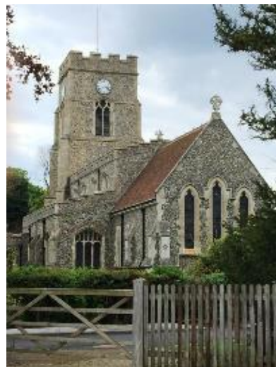
Church tower for mast? - E Clarke
