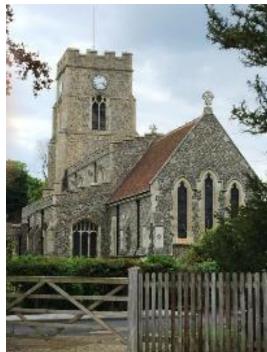
Church tower for mast? - E Clarke
