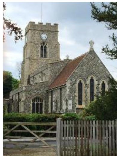
Church tower for mast? - E Clarke
